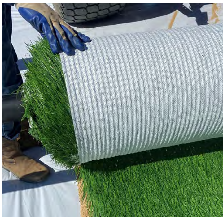
Fig 39. Hybrid turf being installed
