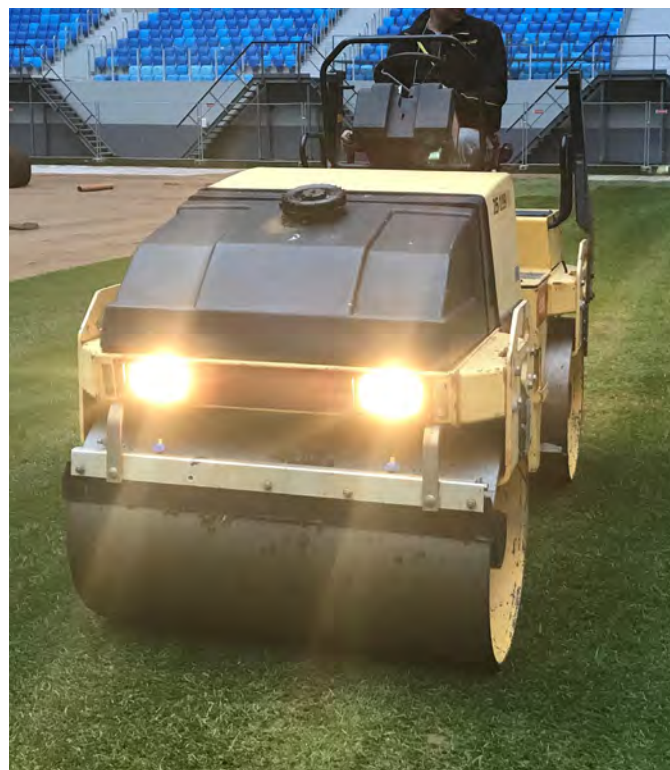
Fig 21. Rolling newly installed sod
