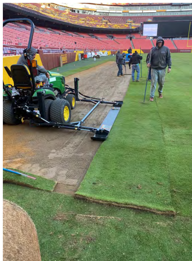
Fig. 20. Post sod install joint pushing using specialist machine
