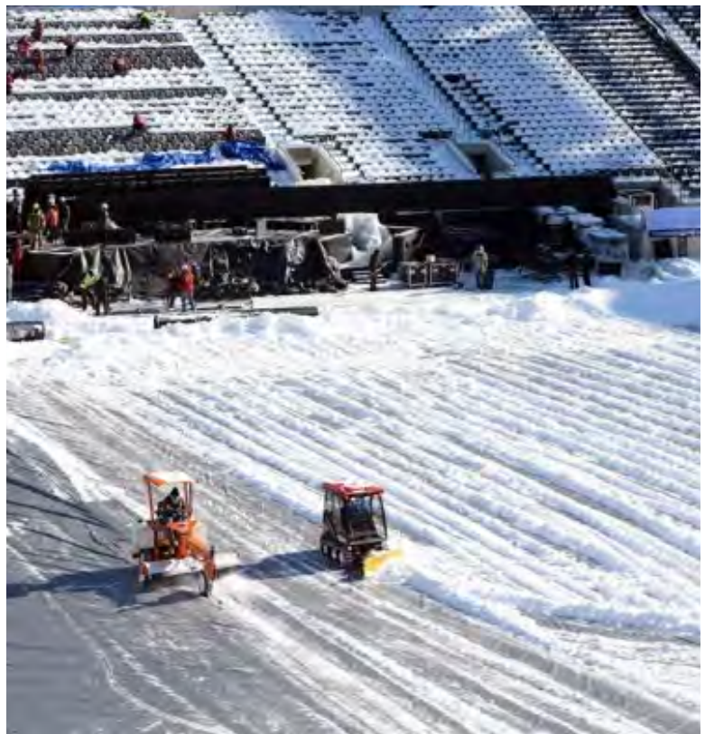
Fig 56. Field tarp cover in place (top) and snow plowing off field (bottom)
