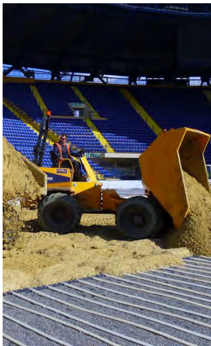
Fig 7. Placing rootzone over heating pipes
