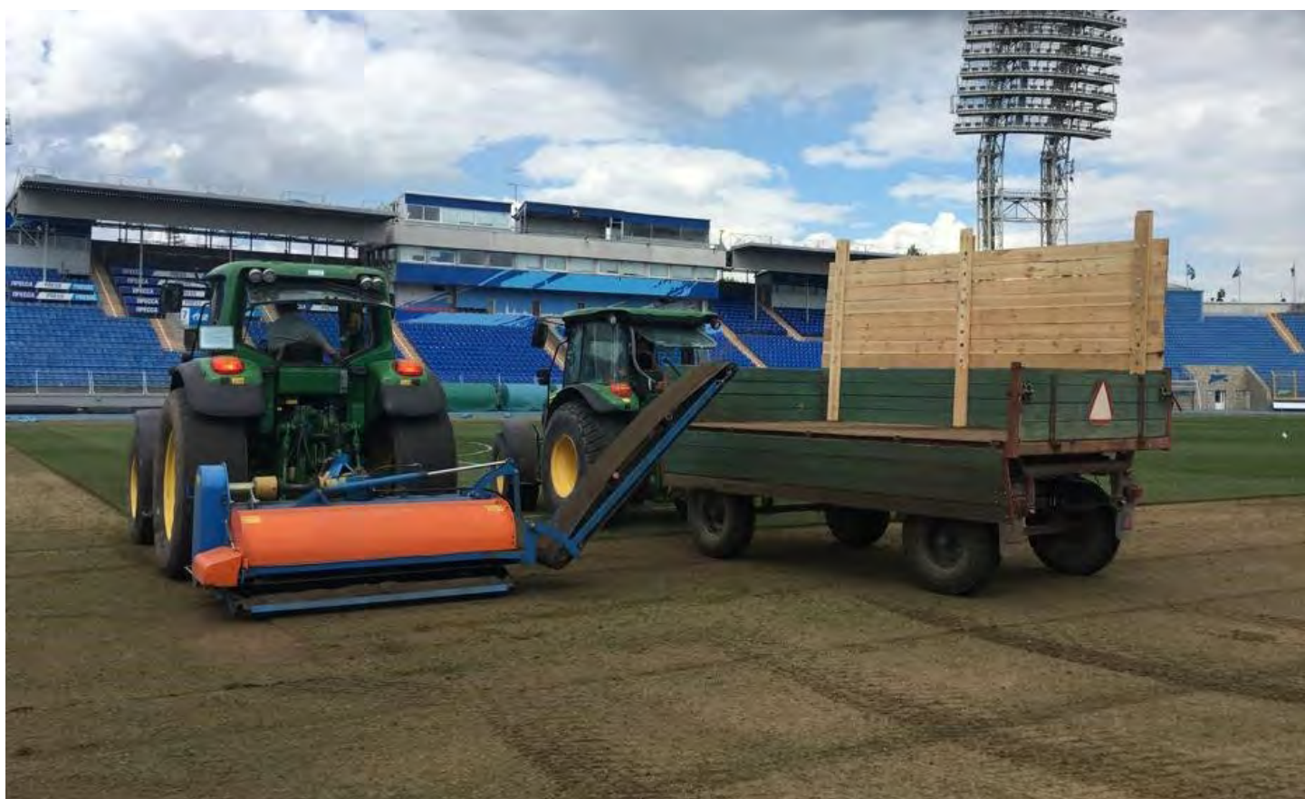
Fig 18. Sod removal with specialized equipment
