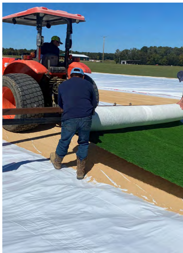
Fig 38. Installation of hybrid carpet at sod farm
