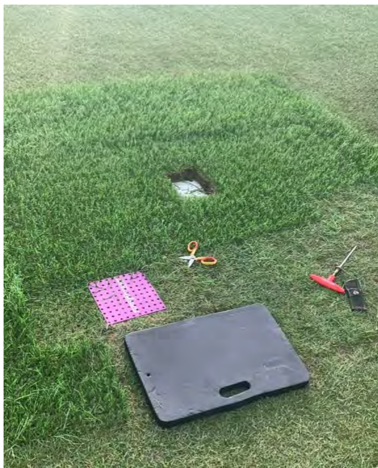
Fig 42. Hand stitching repair of hybrid stitched grass
