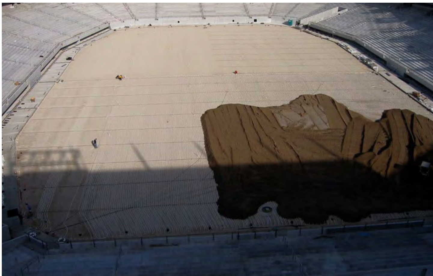
Fig 6. Rootzone installation
