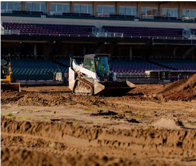
Fig 2. Field subbase construction
