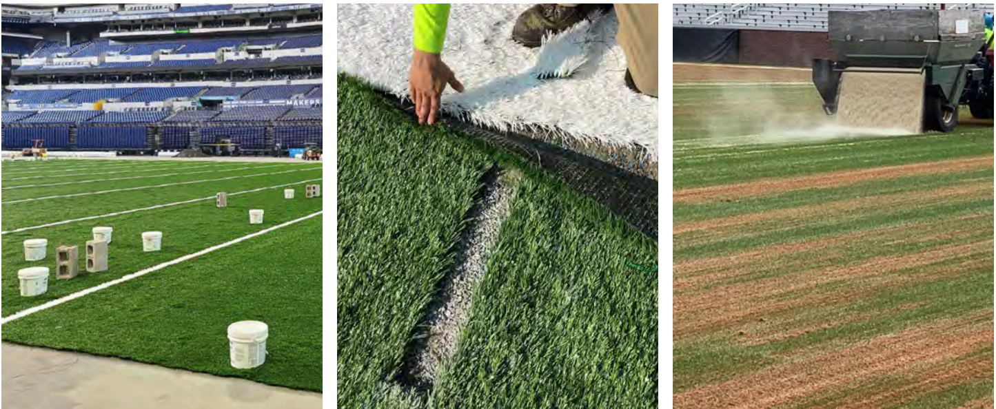
Fig. 49. Panel layout and alignment (left), inlaying field markings (center), and infill spreading (right)
