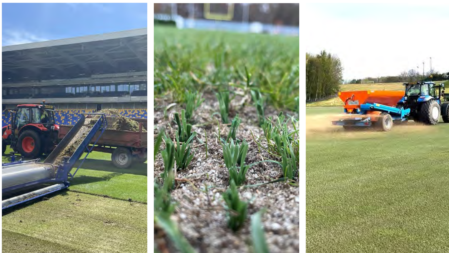
Fig 41. Sand topdressing before seeding (left), fibers left upstanding (middle) and vegetation removal during renovation (right)
