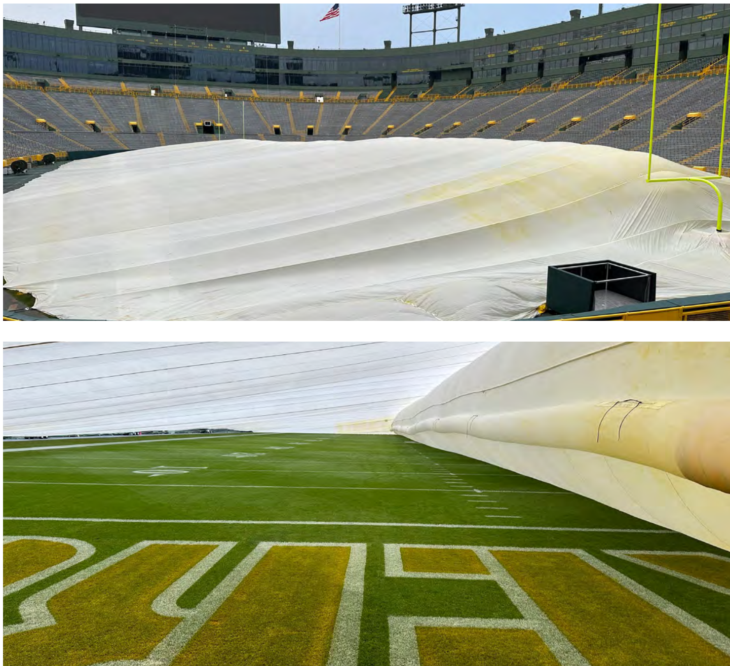
Fig 27. Suspended tent style field cover. View from the stands (top) and from inside the cover (bottom)
