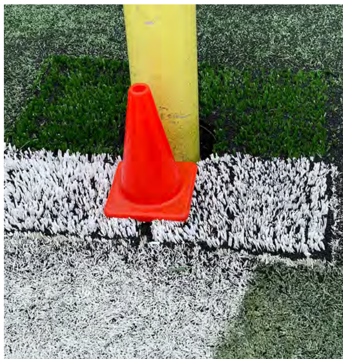
Fig. 52. Synthetic turf installed over and adhered to box cover
