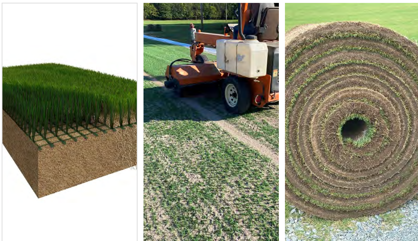
Fig 37. Hybrid grass concept (left), sand filling and installation (middle) and harvested rolled hybrid carpet grass (right)
