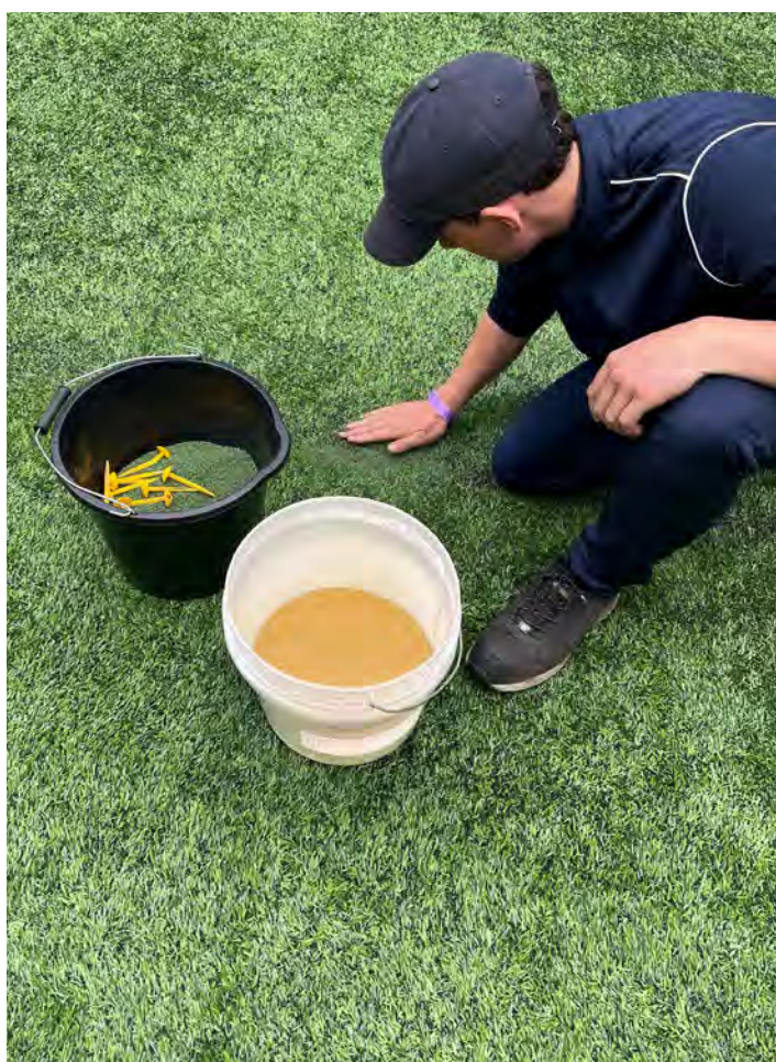
Fig. 57. Adding infill to low areas (left); example of objective testing to inform remediations (right)
